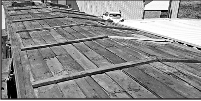
The bare car roof with a minor repair where a hole had been cut for a stack. – Photo © 2017 Duane Danielson.
