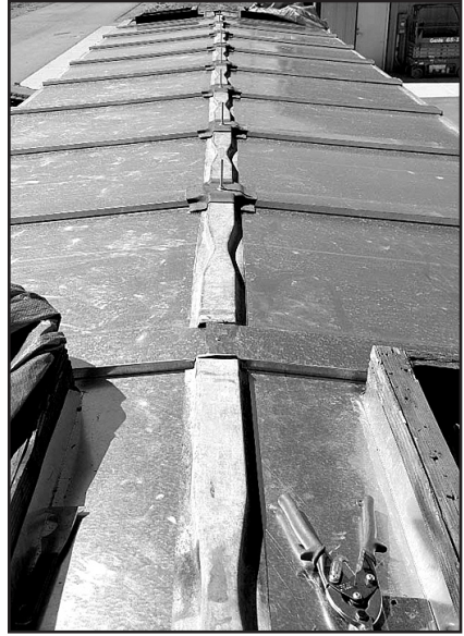
New galvanized roof panels and seam covers fabricated and installed by Holt Sheet Metal. The old ridge pieces were reused. – Photo © 2017 Duane Danielson.
